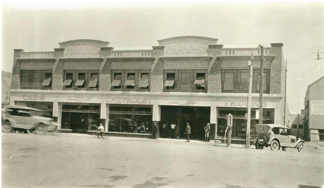
State Library of South Australia - Franklin Street, Adelaide, South Side [B 2444]. Acre 264 Franklin Street, Adelaide, south side. Photographed on January 27, 1925, soon after its completion. The confidence expressed by the new Mann's Motors' building reflects the growing popularity of the motor car. The car by the bowsers is a Chevrolet tourer, 21.7 horsepower, registration number 38420, owned by Mann's. The left side of the building is 25 yards east of Young Street. Frontage is 31 yards. For a photo of Mann's staff, see B 24452. Approximately 1925. Photographer, State Library of South Australia. Part of Acre 264 Collection.
